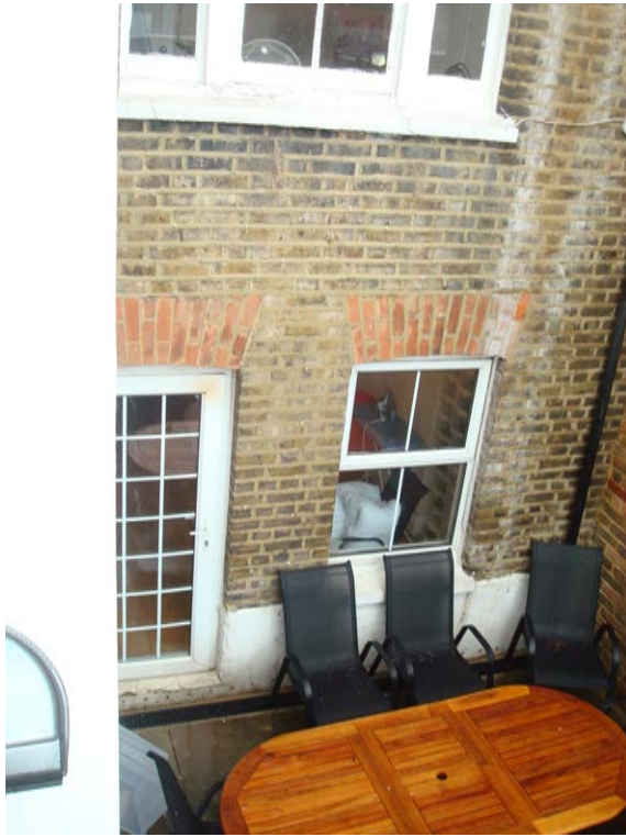
Lower Ground View
