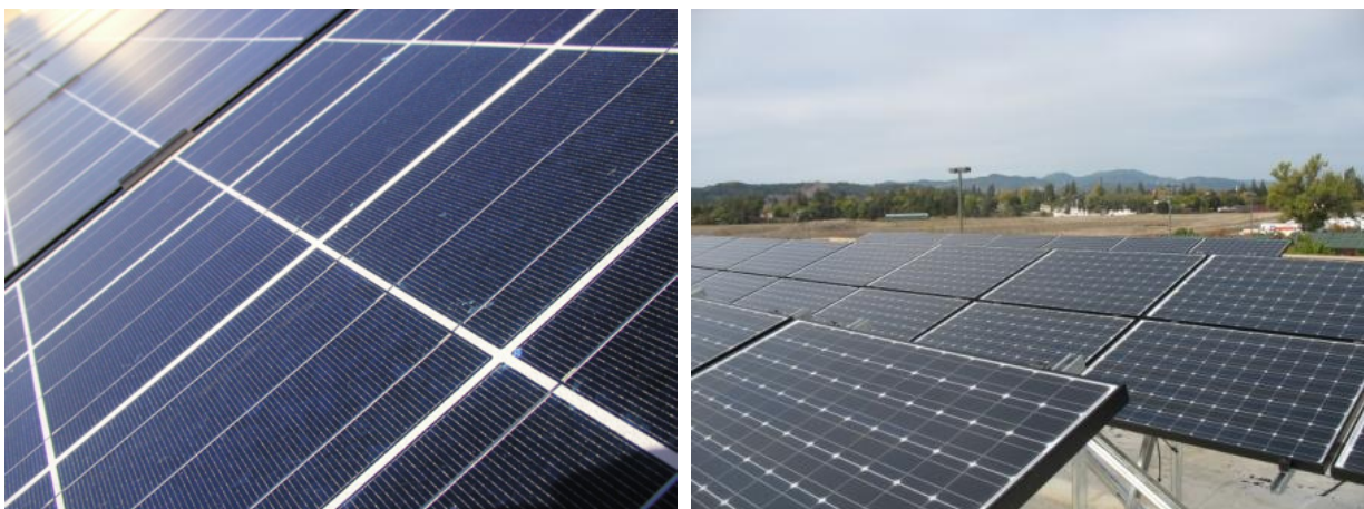
Figure 4 - Typical photovoltaic panel installations
