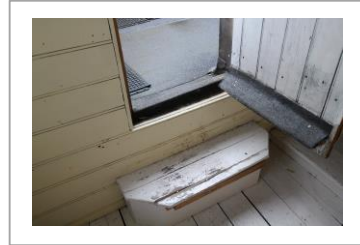
Roof terrace and threshold
