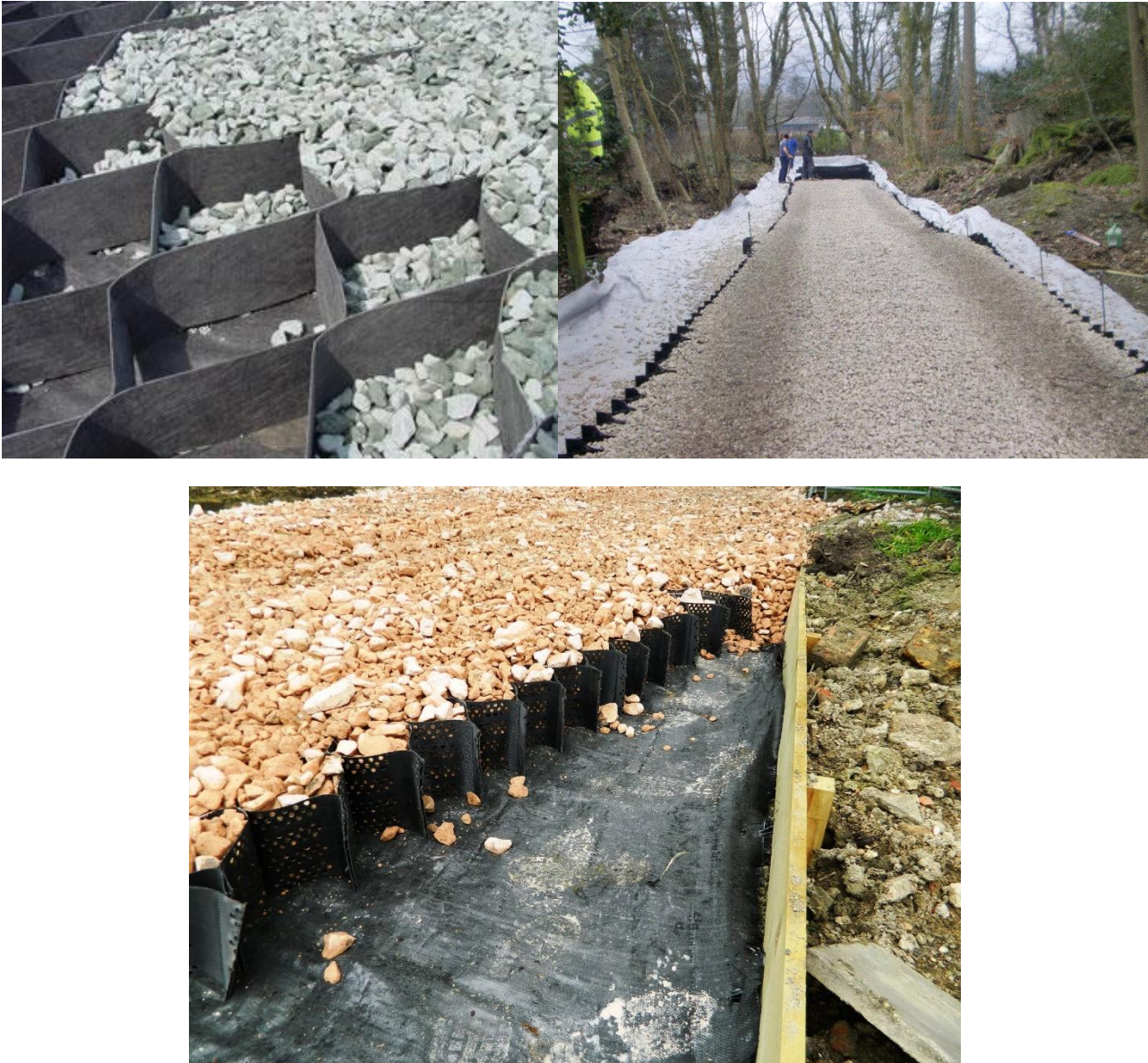
Figure 7. Photographs illustrating cellular confinement system used to form an above-ground no-dig driveway
