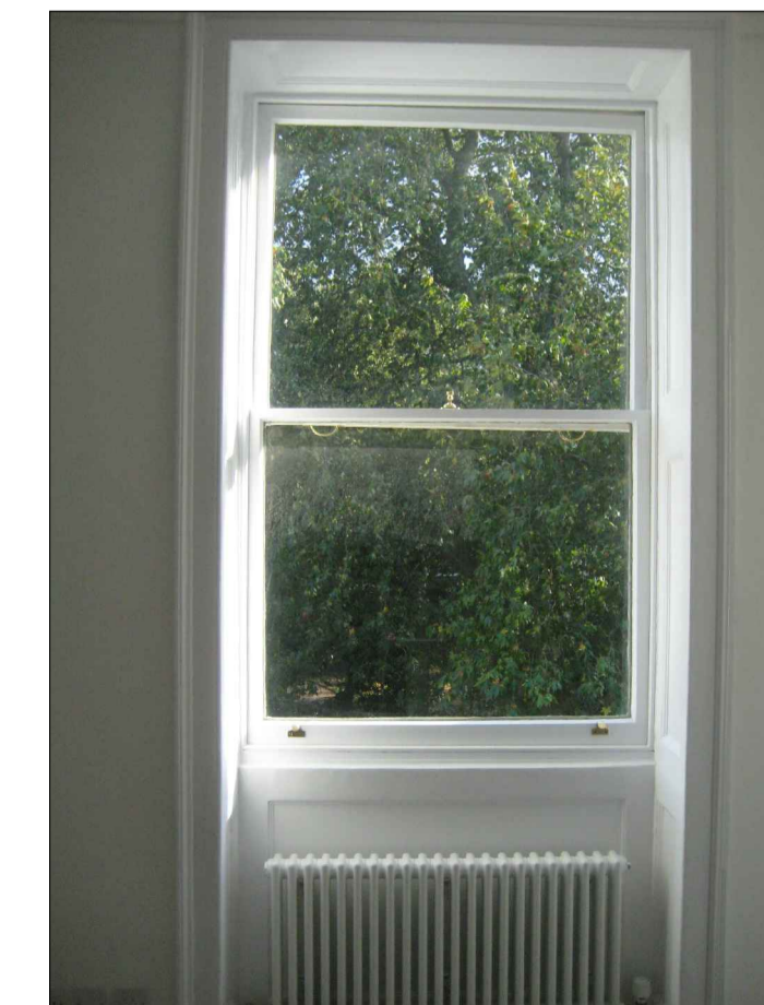
INTERNAL PHOTOGRAPH EXISTING WINDOW W15.S03
