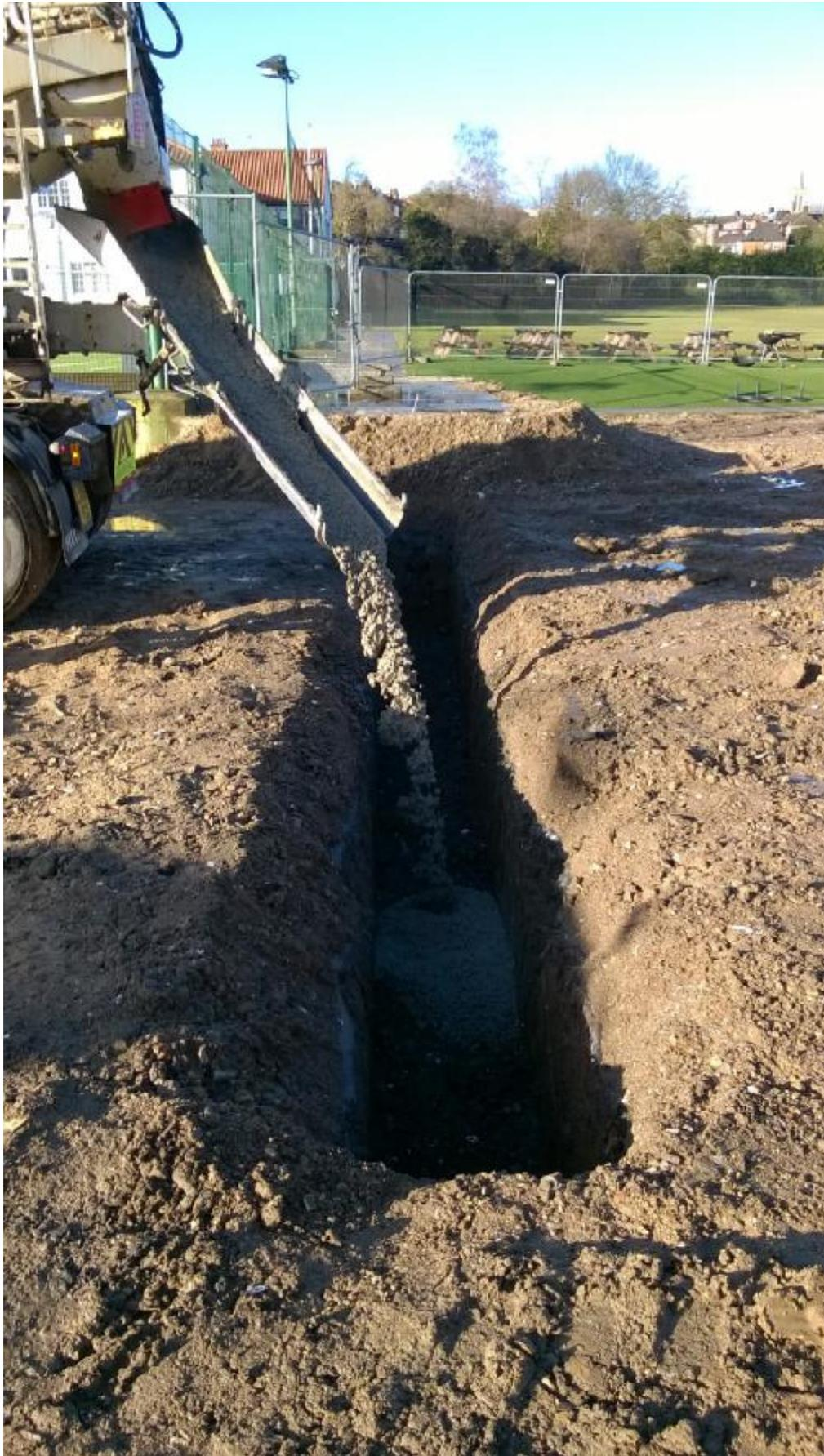
29/1/2015 Concrete to foundation complete and showing water main laid to foundation.
