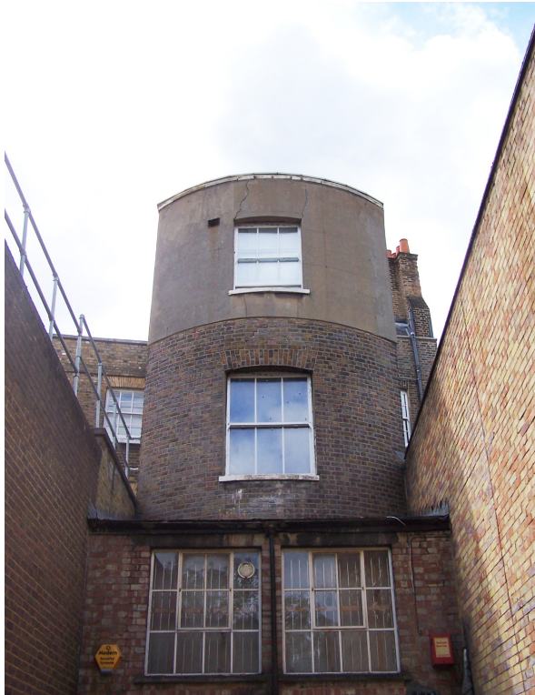
Rear View - Existing
