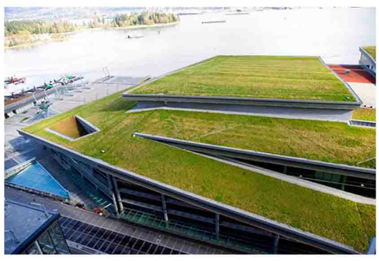
Extensive Green Roof
