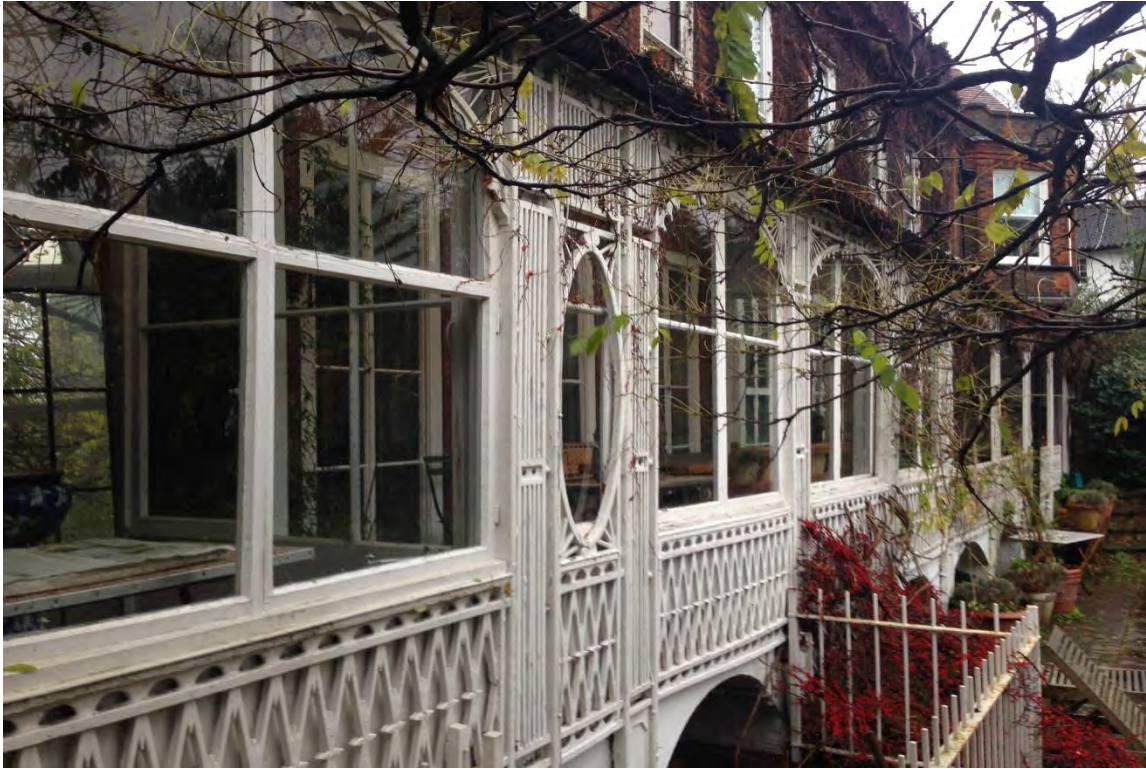
View of existing house conservatory to terrace
