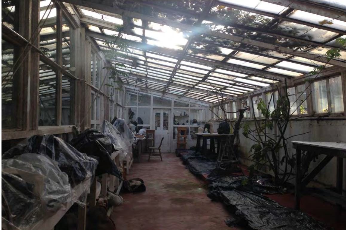
Internal view of existing orangery
