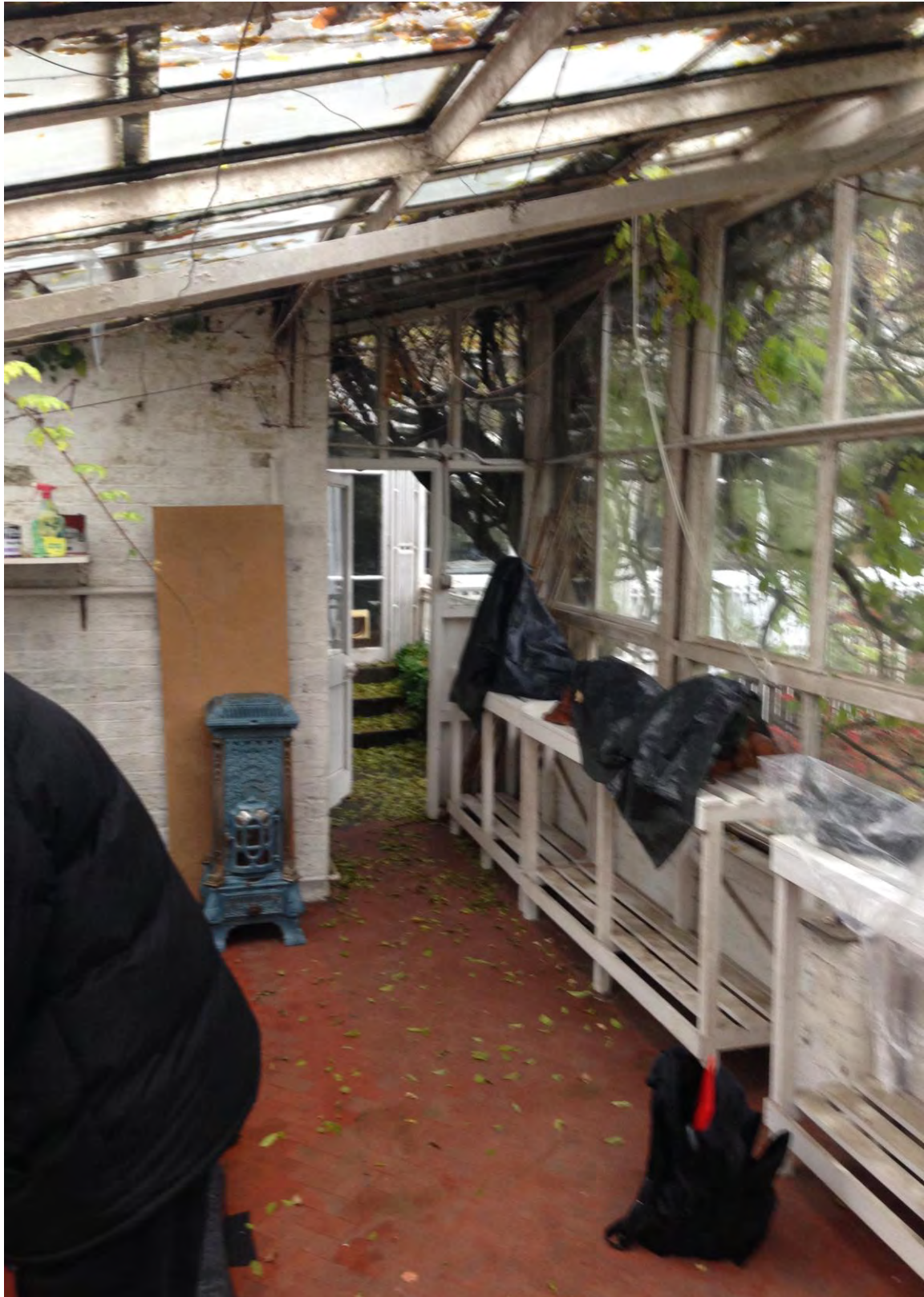
Internal view of Orangery entrance facing onto house and garden area – Currently disconnected solid fuel floor mounted stove in background to be relocated in new garden room
