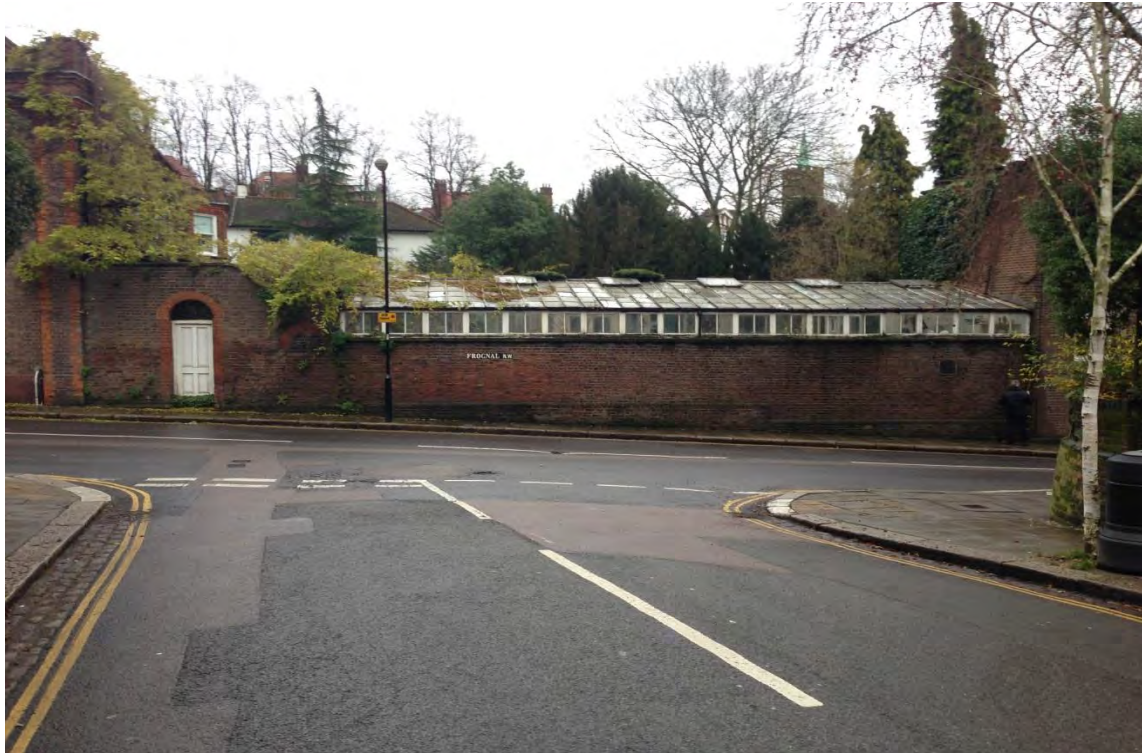
View of existing orangery from road
