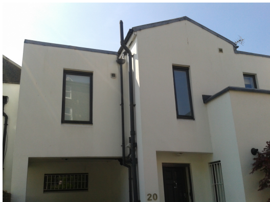
Fig.3 - Image showing small ground floor window recessed under first floor projection.
