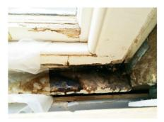
It is, therefore, proposed as part of this application to replace these windows. The new windows would be like for like replacements. They would be timber painted, single glazed, sash windows.
