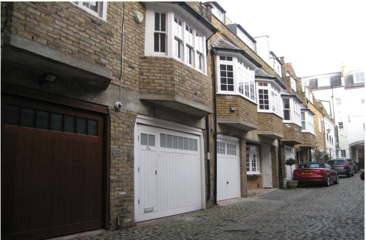
View showing variation of façades treatment along the same row
