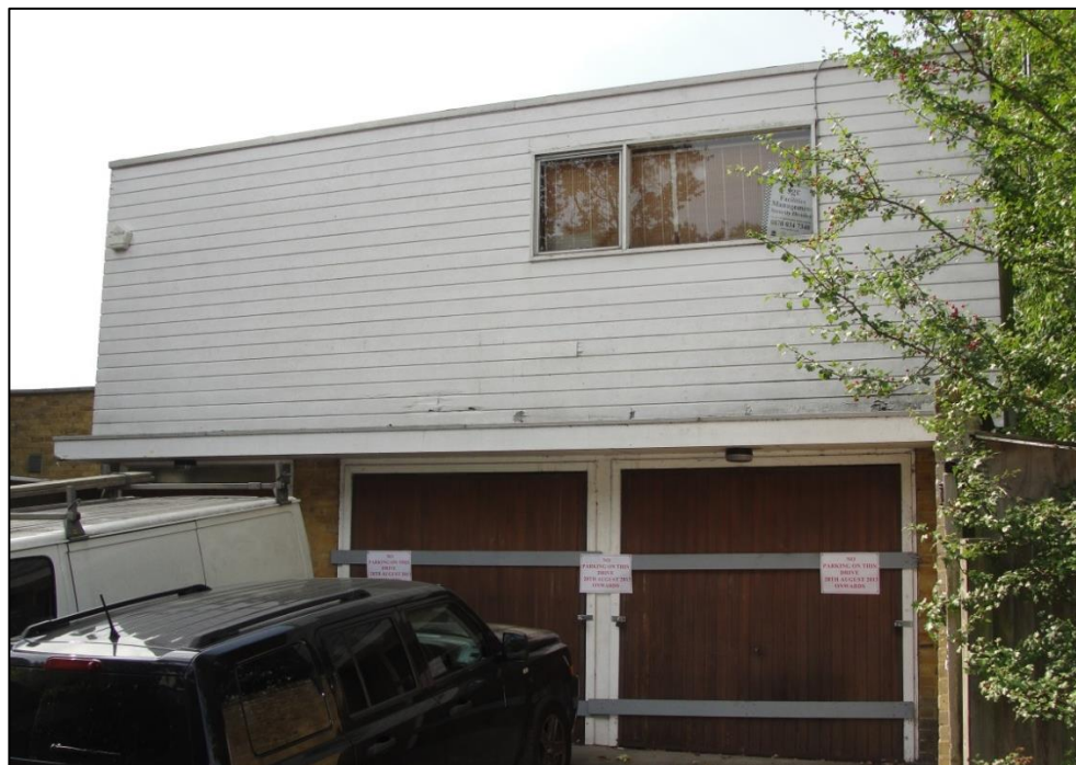
Photograph 2.1: View of the front elevation looking west from Fitzroy Park.
