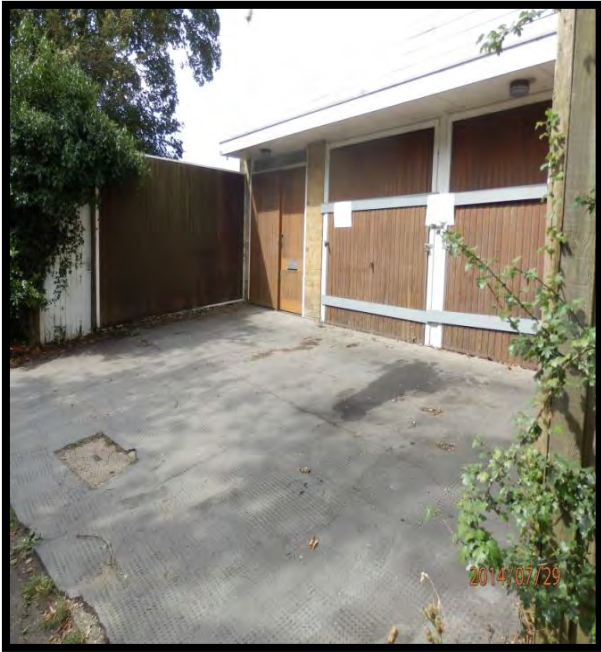
Existing drive in front of double garages
