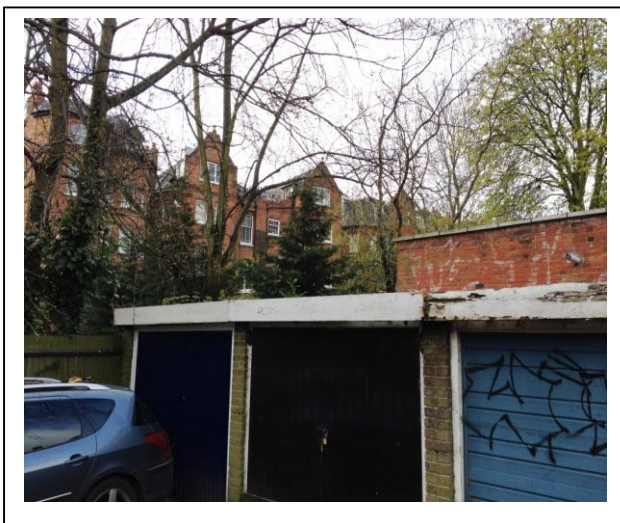
View of Garage
