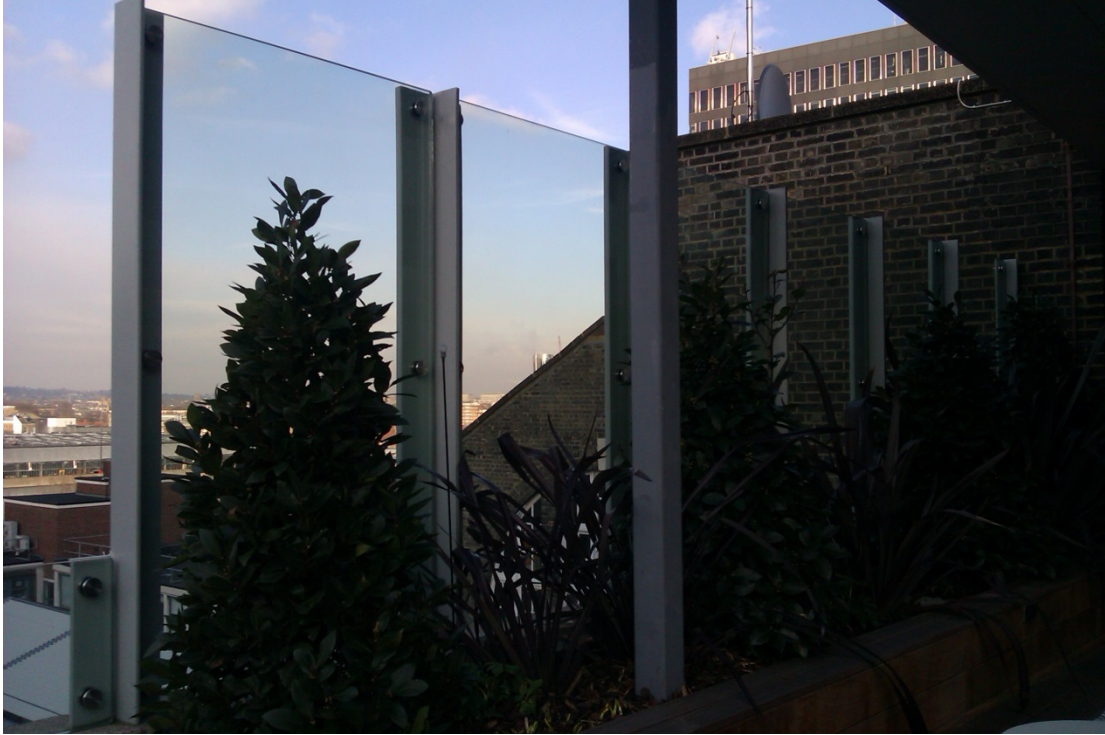
Image 02: existing adjacent 170cm high glazed barrier to be retained
