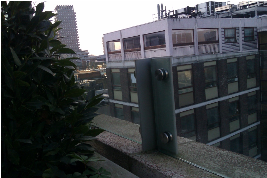
Image 01: existing 38cm high safety barrier to be replaced
