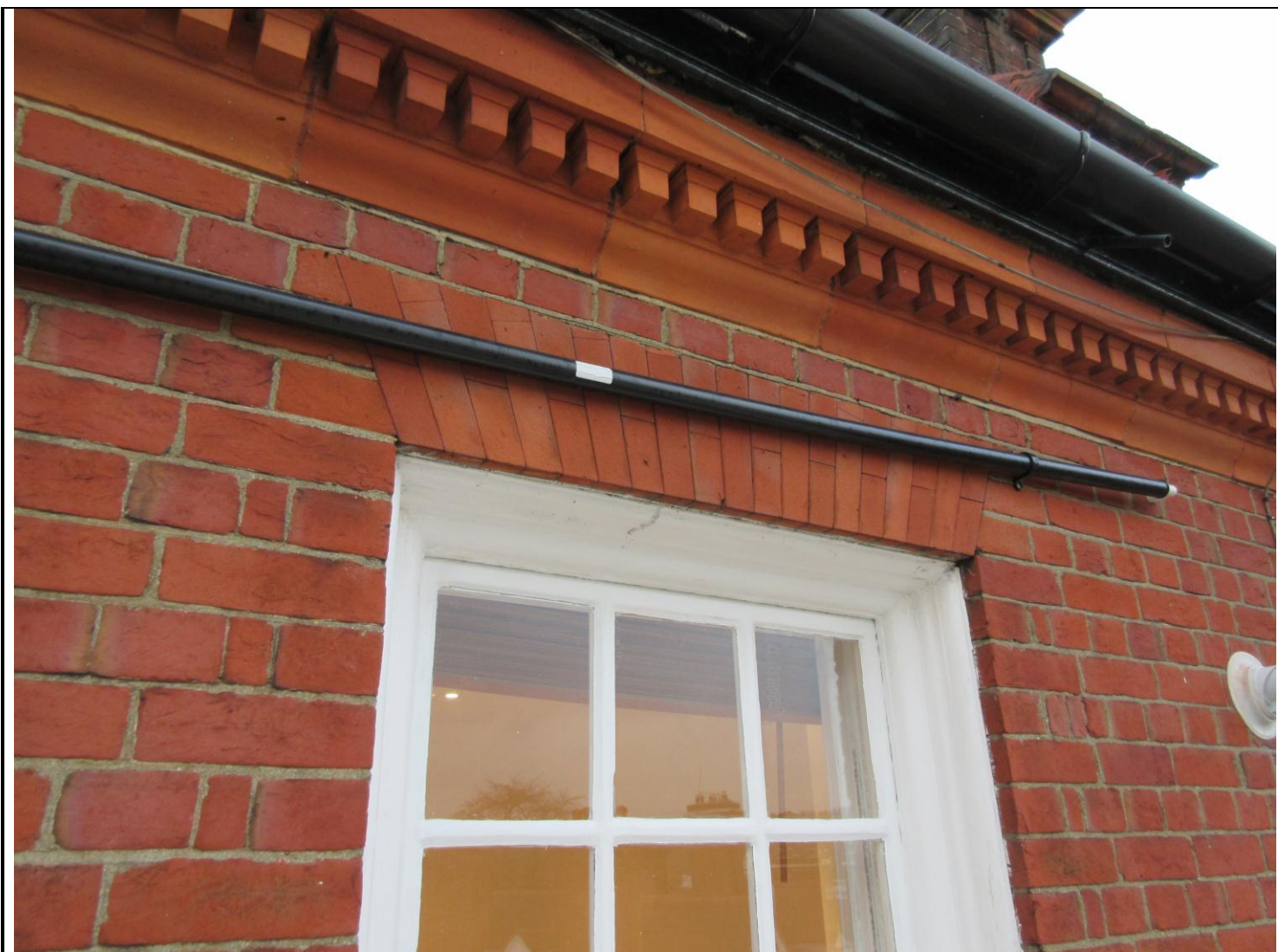
Detailed rubbed brick door and window heads
