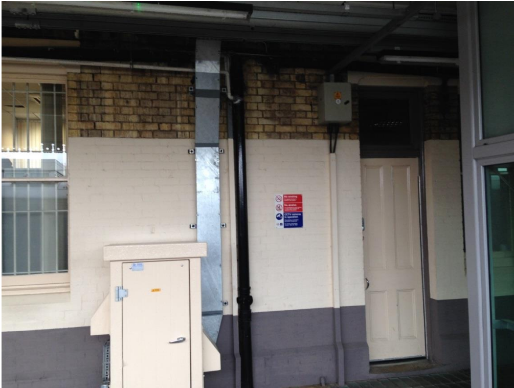
Plate 11: Showing the plastic rainwater downpipe on the northern elevation of the Premises adjoining the southern platform of the station.
