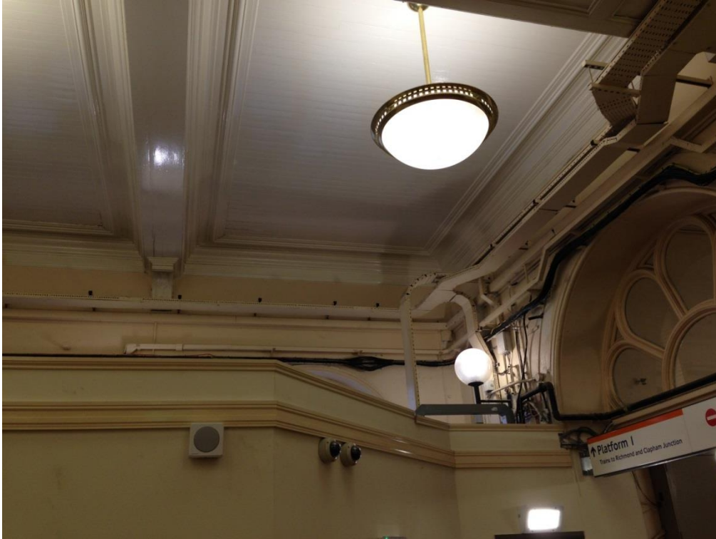
PLATE 3: Showing the south-western corner of the Booking Hall. The proposed downpipe location will be to the right, adjoining the corner. The existing tongue and groove timber boards forming part of each coffered ceiling section are clearly visible above.
