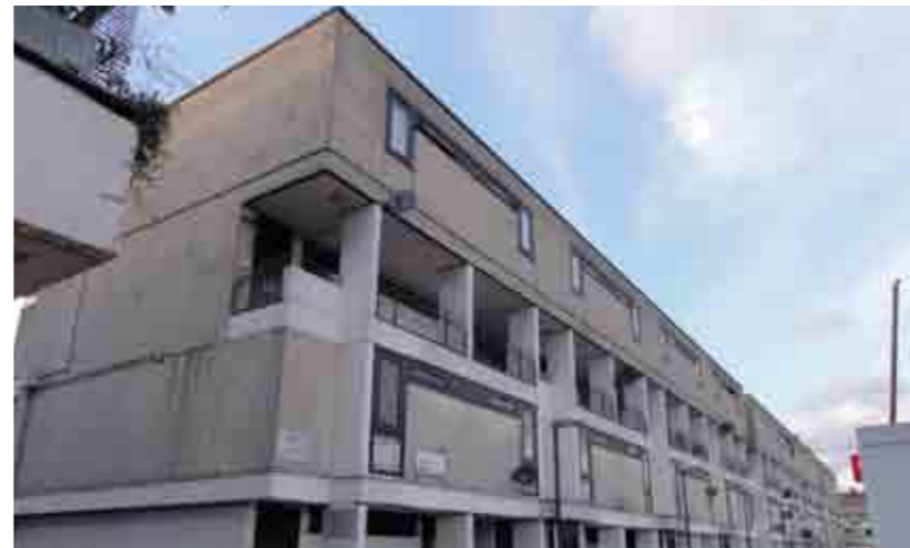
Existing Broadfield Lane Block
