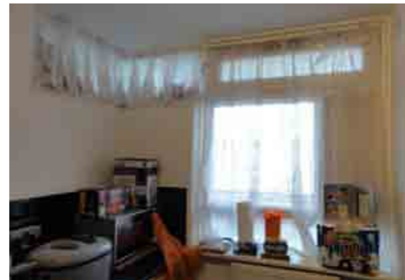
Above: Kitchen window with solid timber opening panel
