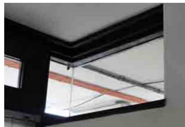
Above: Corner glazing detail to the kitchen
