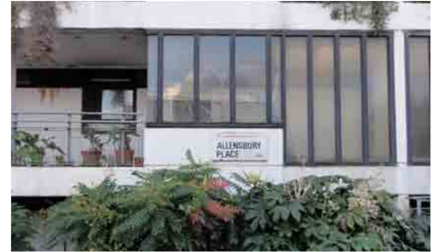
Existing Allensbury Place Block Fenestration
