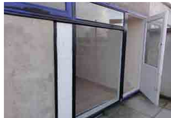
Above: External west facade glazing with timber panel
