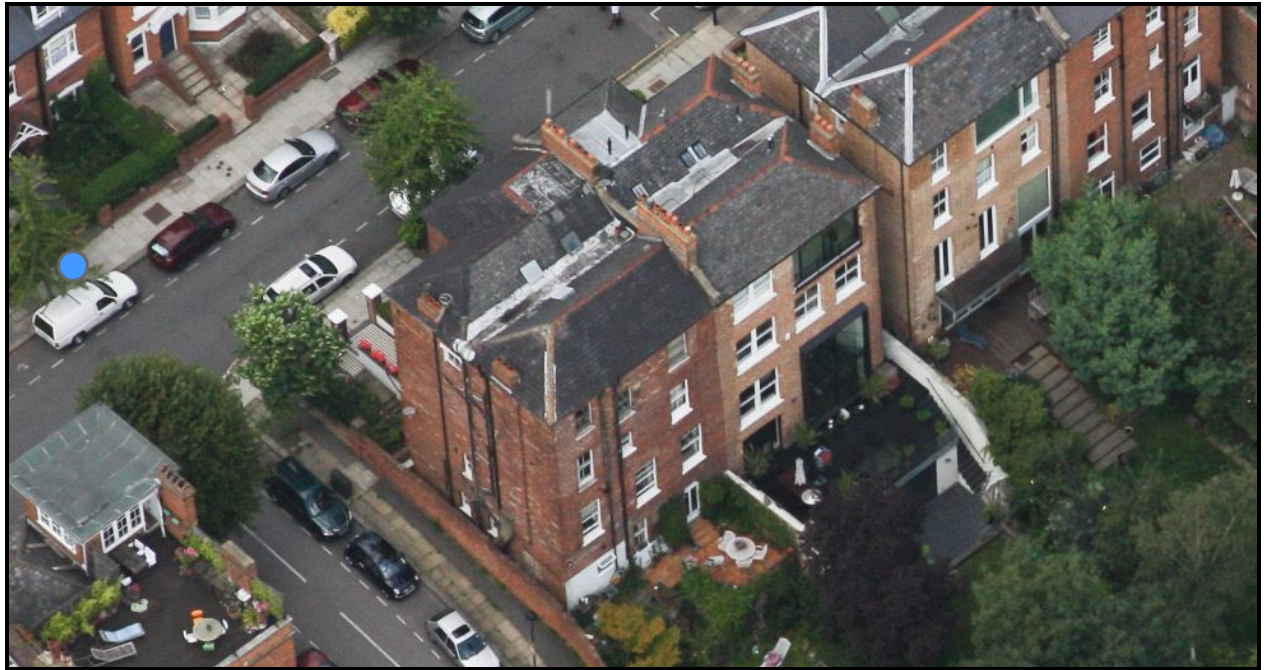
Photo 1- Aerial view showing double valley roof
