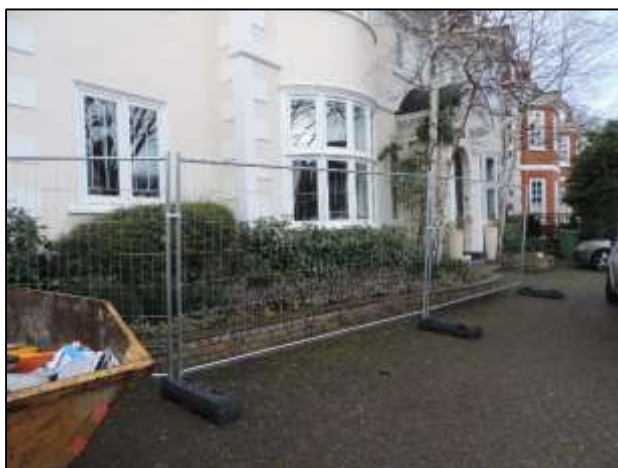
Photo 1: Tree protection barriers at the front of the property
