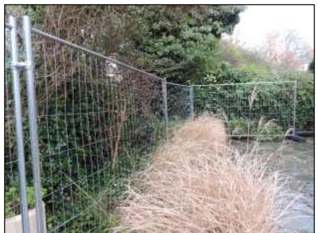
Photo 2: Tree protection barriers at the rear of the property
