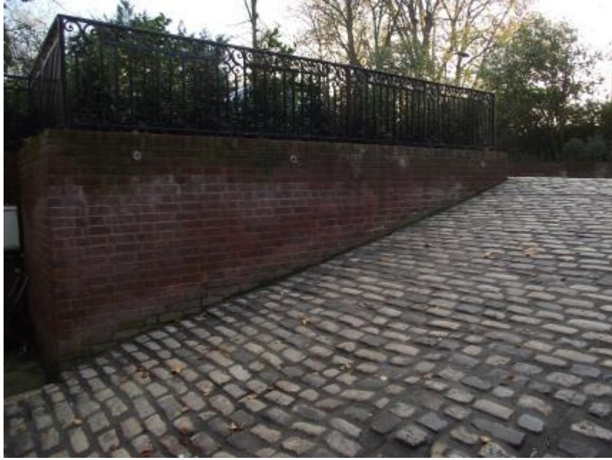
Existing Ramp from garage to parking area
