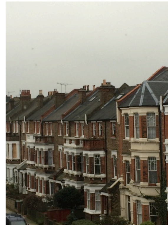
Roof windows installed to nearby properties In Gondar Gardens
