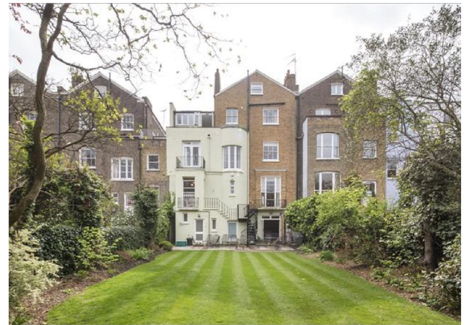
⑥ REAR VIEW 54 REGENT'S PARK ROAD WITH No.52 ON LEFT & No.56 ON RIGHT
