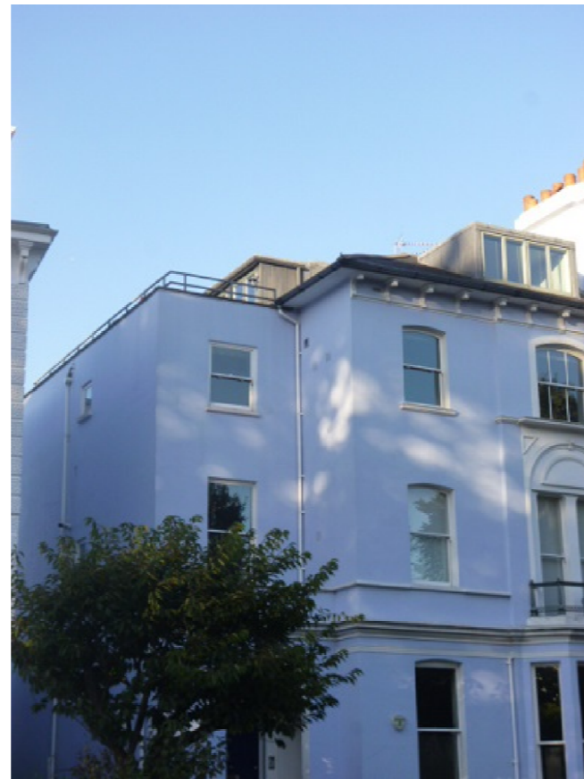
② VIEW OF SIDE WING FROM STREET 56 REGENT'S PARK ROAD
