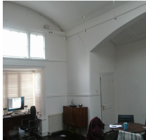
Interior of main room looking towards the front entrance
