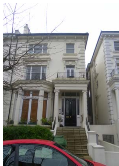
Terrace with balustrade & French doors: No 9 Belsize Square
