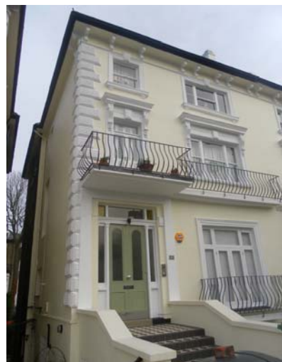
Terrace with balustrade & French doors: No 40 Belsize Square
