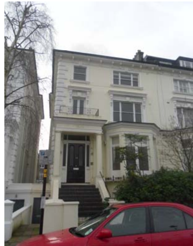
Terrace with balustrade & French doors: No 14 Belsize Square
