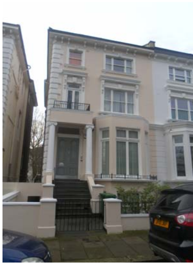
Terrace with balustrade & French doors: No 2 Belsize Square
