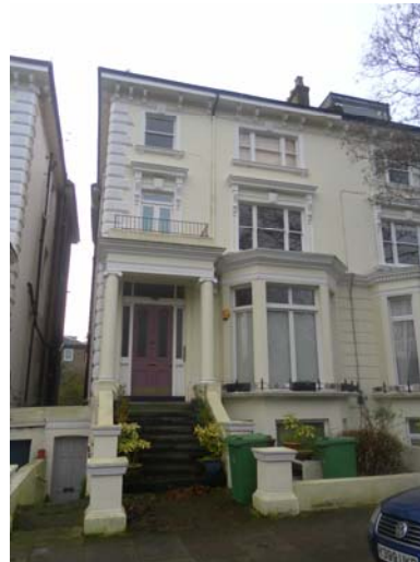
Terrace with balustrade & French doors: No 6 Belsize Square
