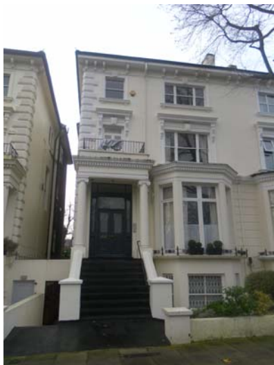
Terrace with balustrade & French doors: No 8 Belsize Square
