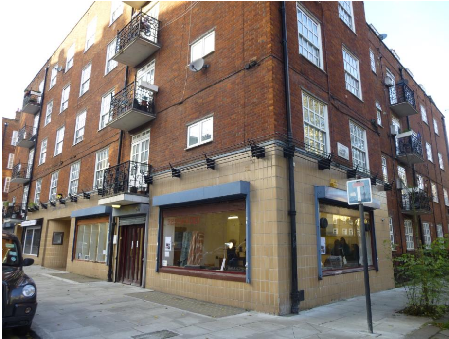
74-76 Cromer Street view from front showing double frontage and residential above and behind
