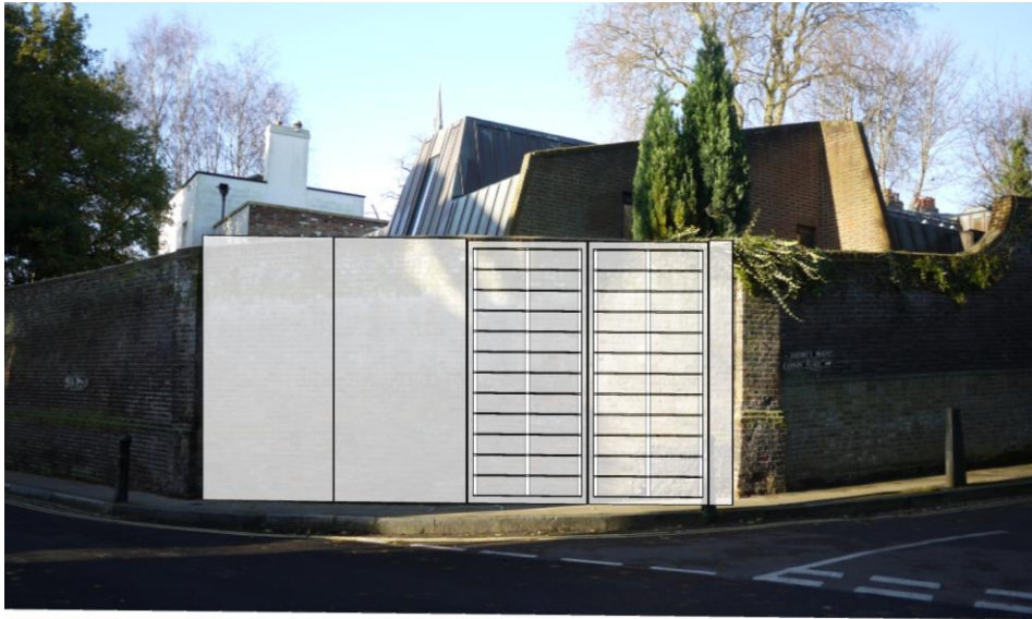
Image showing area of wall to be dismantled with temporary secure hoarding and gates constructed.
