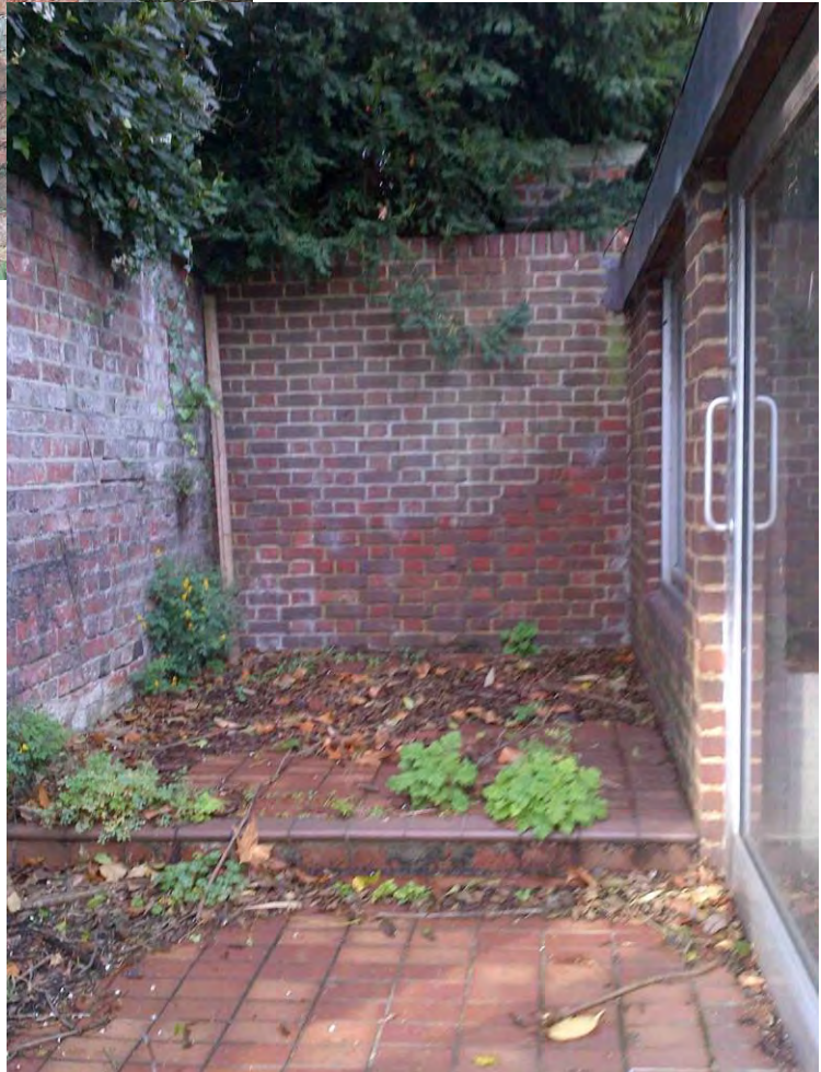
Photo 8: Eastern part of rear retaining wall. Note the more modern brickwork compared with the retaining wall to the west. During the Ground Investigation, TP3 revealed different foundations beneath this section of the retaining wall, compared with the foundations described beneath the rest of the rear retaining wall, indicating it was constructed at a later date. Annex on right.
