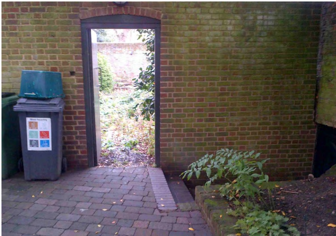
Photo 4: Entrance doorway in the southern part of the western boundary wall. Note the adjacent flight of steps which lead up from the Well Road footway, and the more modern brickwork of the western boundary wall compared with the southern and eastern boundaries.
