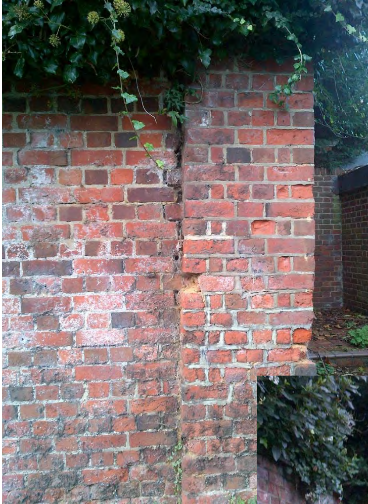
Photo 8: Eastern part of rear retaining wall. Note the more modern brickwork compared with the retaining wall to the west. During the Ground Investigation, TP3 revealed different foundations beneath this section of the retaining wall, compared with the foundations described beneath the rest of the rear retaining wall, indicating it was constructed at a later date. Annex on right.
