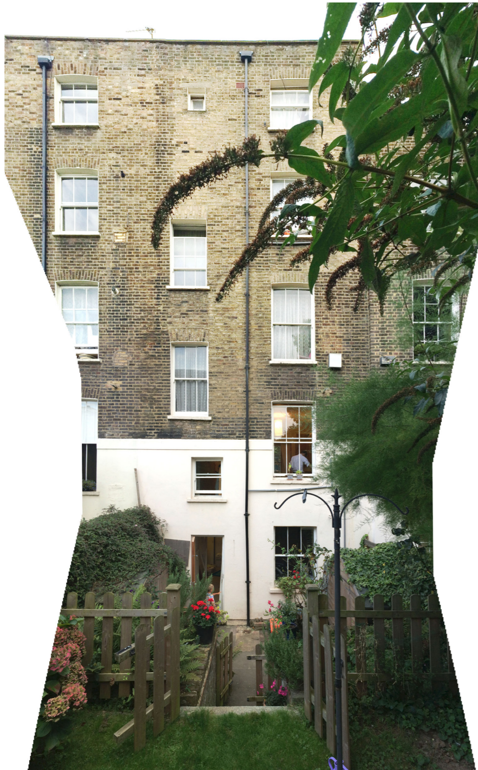
View of rear elevation from upper garden - existing
