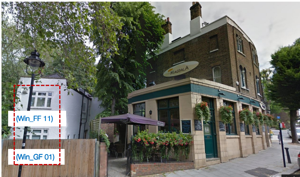
Figure 2-3 House 2a South Hill Park Road- Front Elevation
