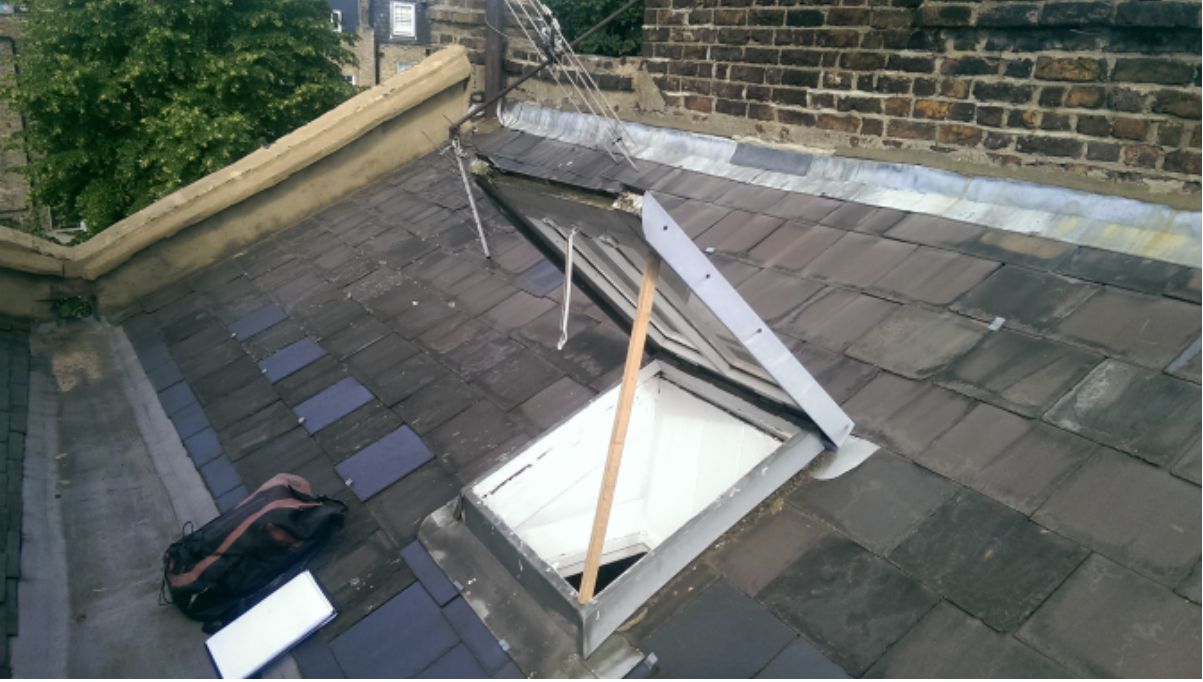
Roof level showing the existing hatch
