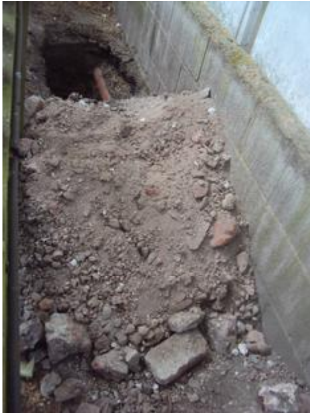
Photograph 21: TP9 – Excavated material
