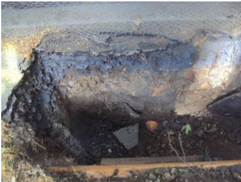
Photograph 12: TP5 – Made ground and 20mm root end
