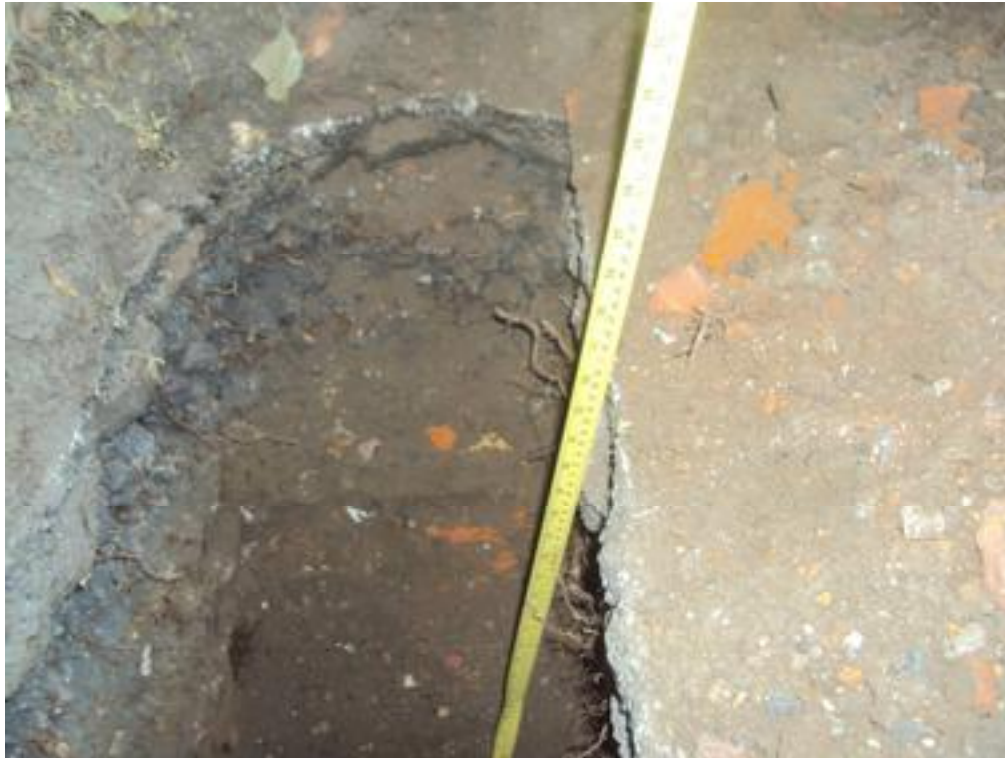
Photograph 15: TP6 – Large root at 600mm depth
