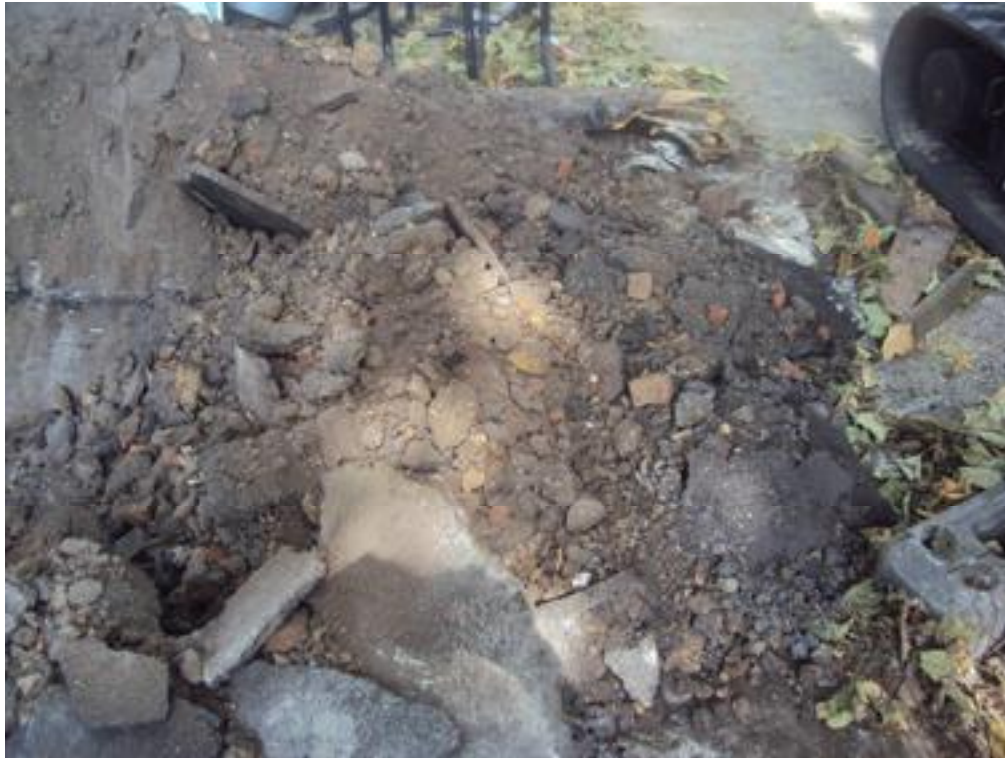
Photograph 9: TP3– Excavated material
