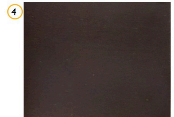
copper 'oxid' cladding to the external columns
