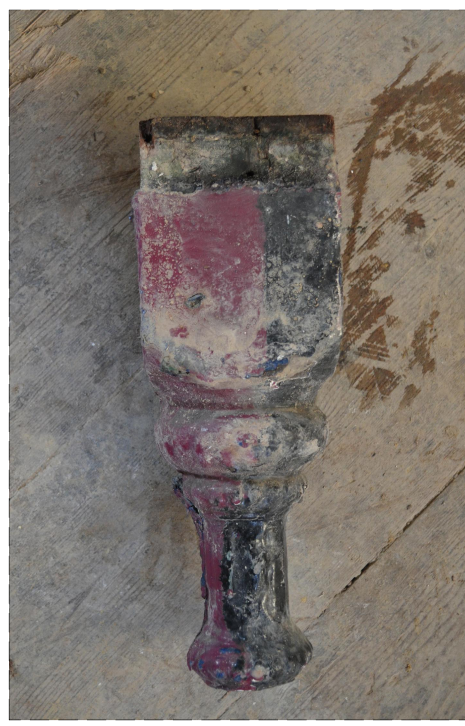
4 1-3 GOODGE STREET SHOP FRONT ORIGINAL CAPPING TO MULLION SCALE: (A1)
