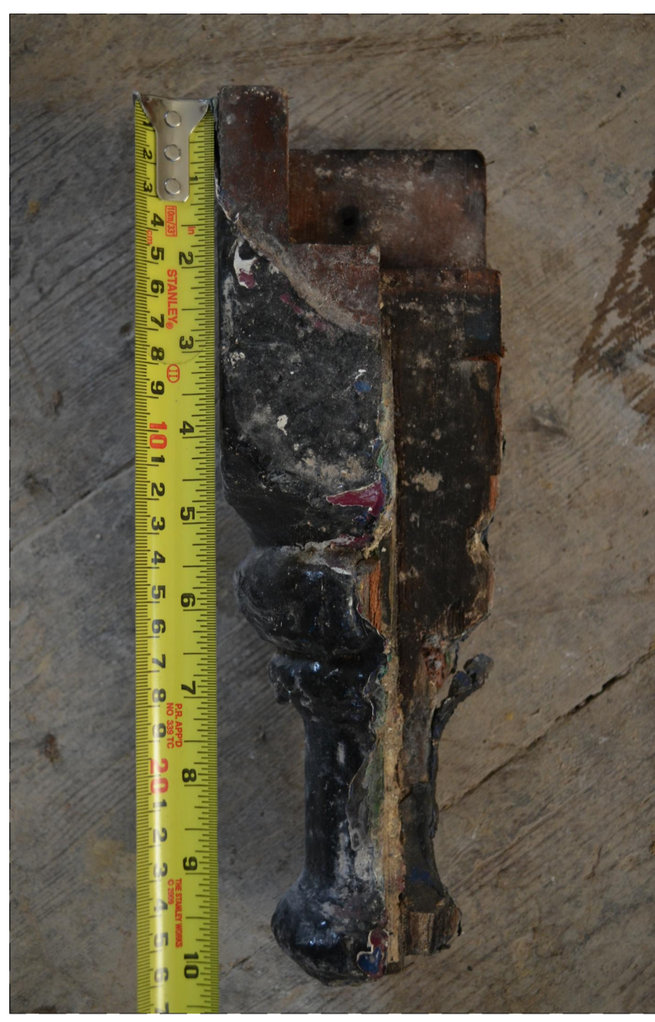
4 1-3 GOODGE STREET SHOP FRONT ORIGINAL CAPPING TO MULLION SCALE: (A1)
