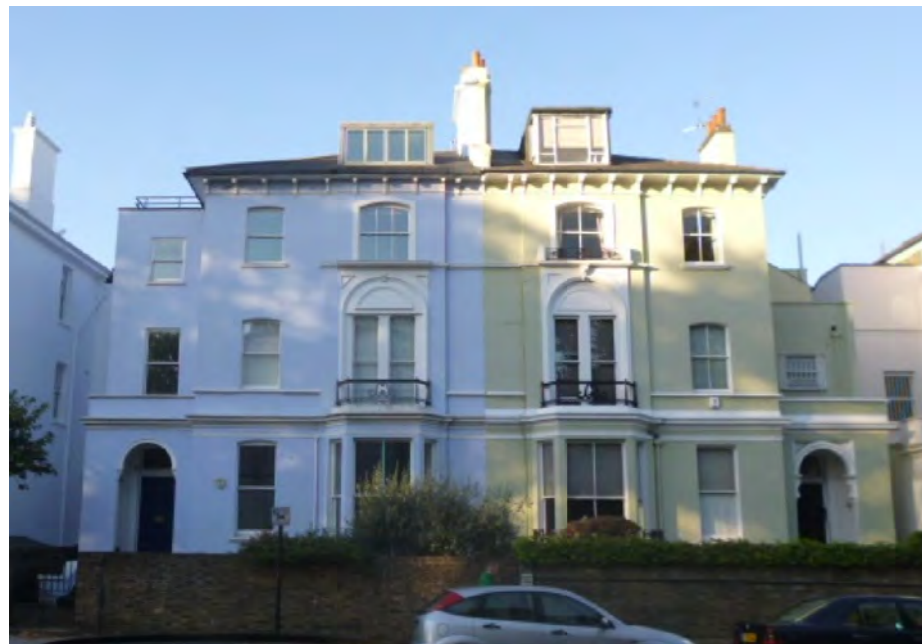
④ FRONT VIEW 54 REGENT'S PARK ROAD WITH No.56 ON LEFT
