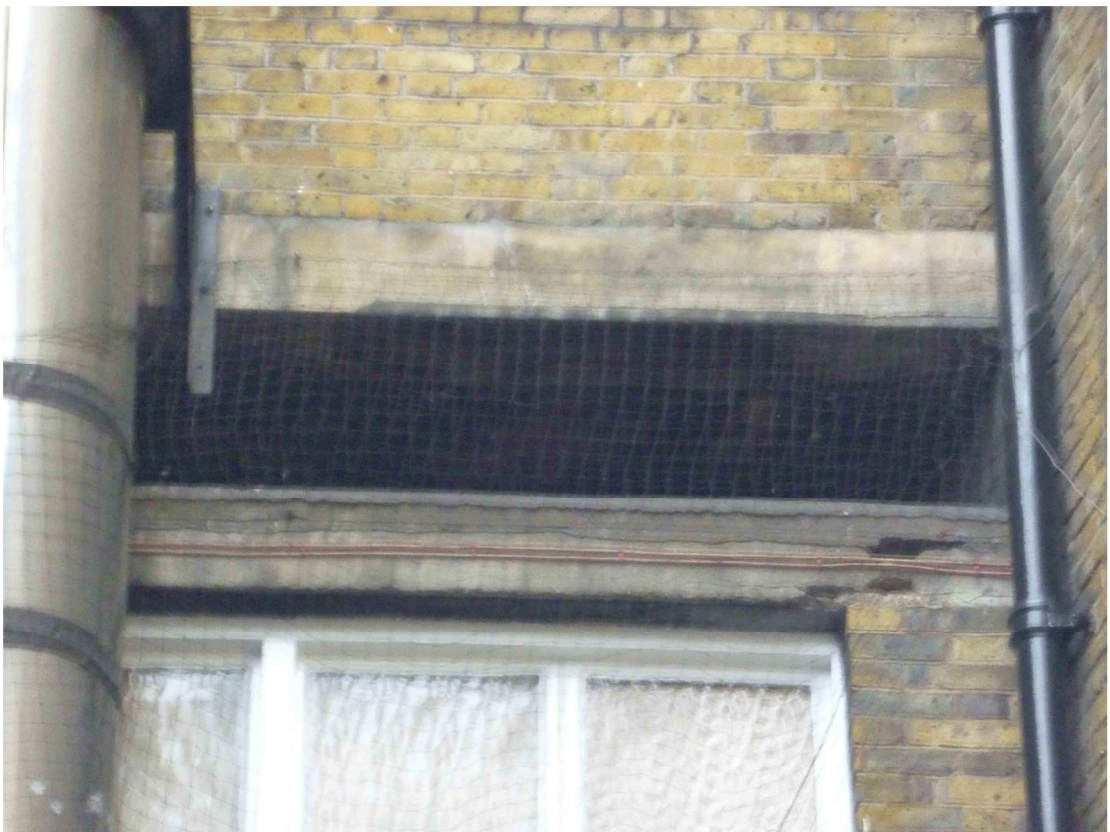
Photo 3 Void between links showing spalling of concrete and bird netting
