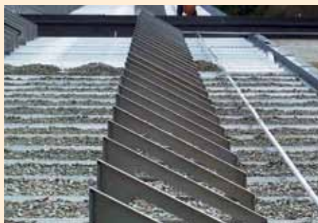
Linking the system with aluminium profiles, for example in a wind zone 2 location, with the adjunct "coast" and unfavourable structural conditions.
