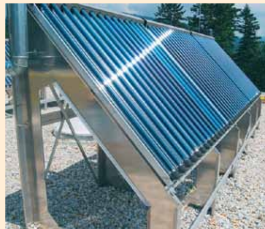
Base frames with a different angle are often used for solar thermal systems.
