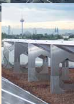
Linking the system with aluminium profiles, for example in a wind zone 2 location, with the adjunct "coast" and unfavourable structural conditions.
