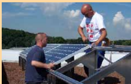
The solar panels are installed.
