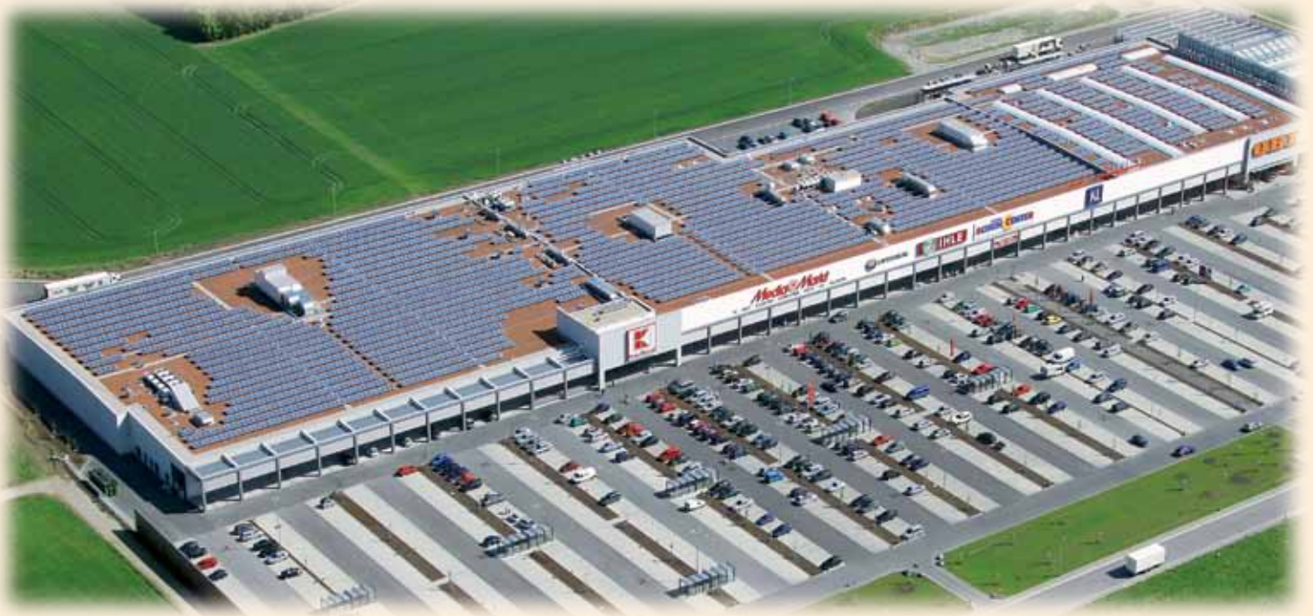
Photovoltaic plant on the roof of the "InCenter" shopping mall in Landsberg/Lech, Germany.
