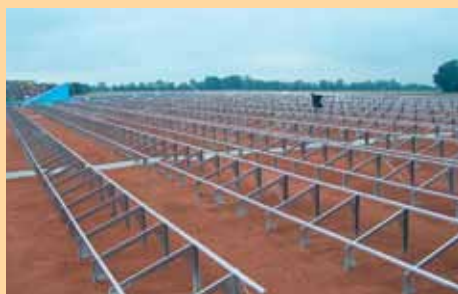
The Solar Base® plates are covered with system substrate as per the required load.
