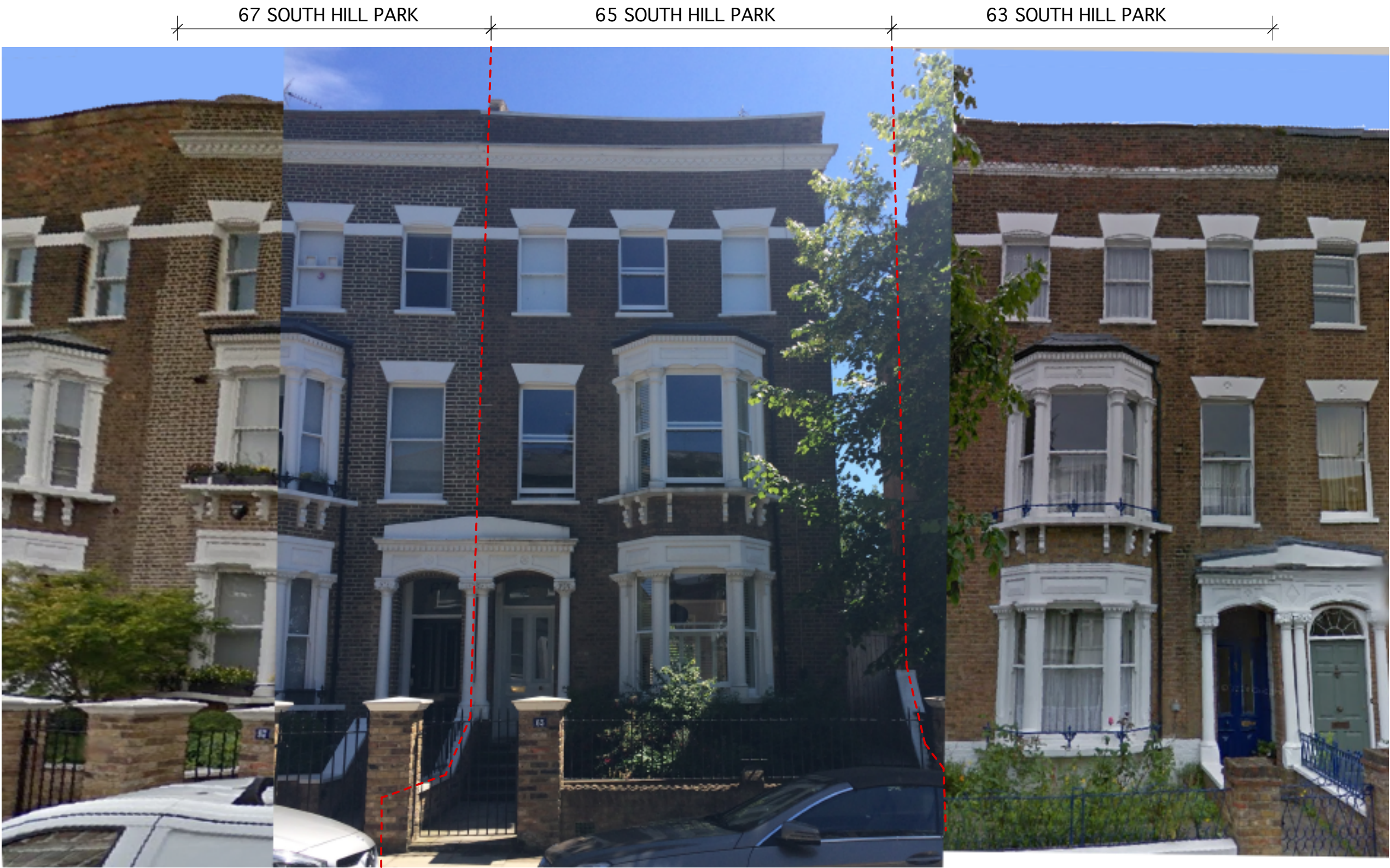
IMAGE 01 - Front Elevation of 65 South Hill Park from public footpath
