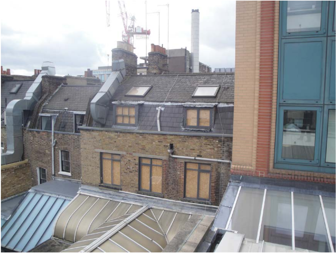
PHOTO 7 ROOF PROFILE OF 74 CHARLOTTE STREET
