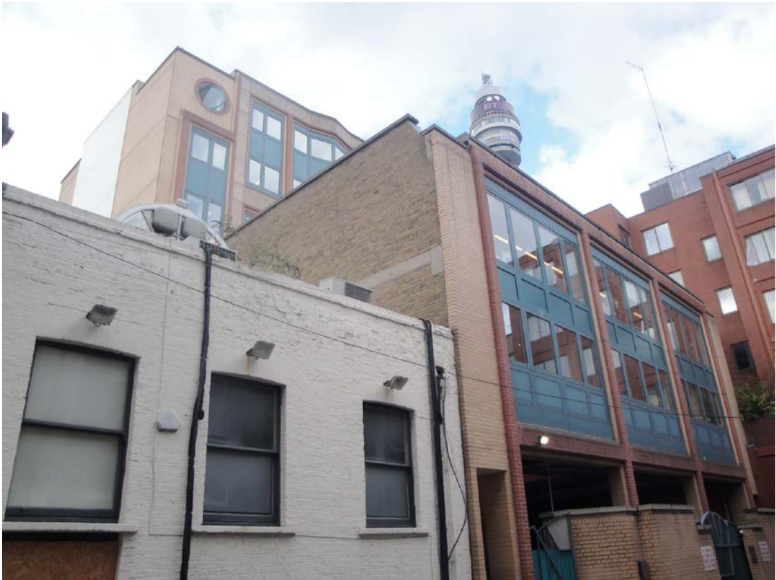
PHOTO 6 REAR OF 74 / 74A CHARLOTTE STREET
