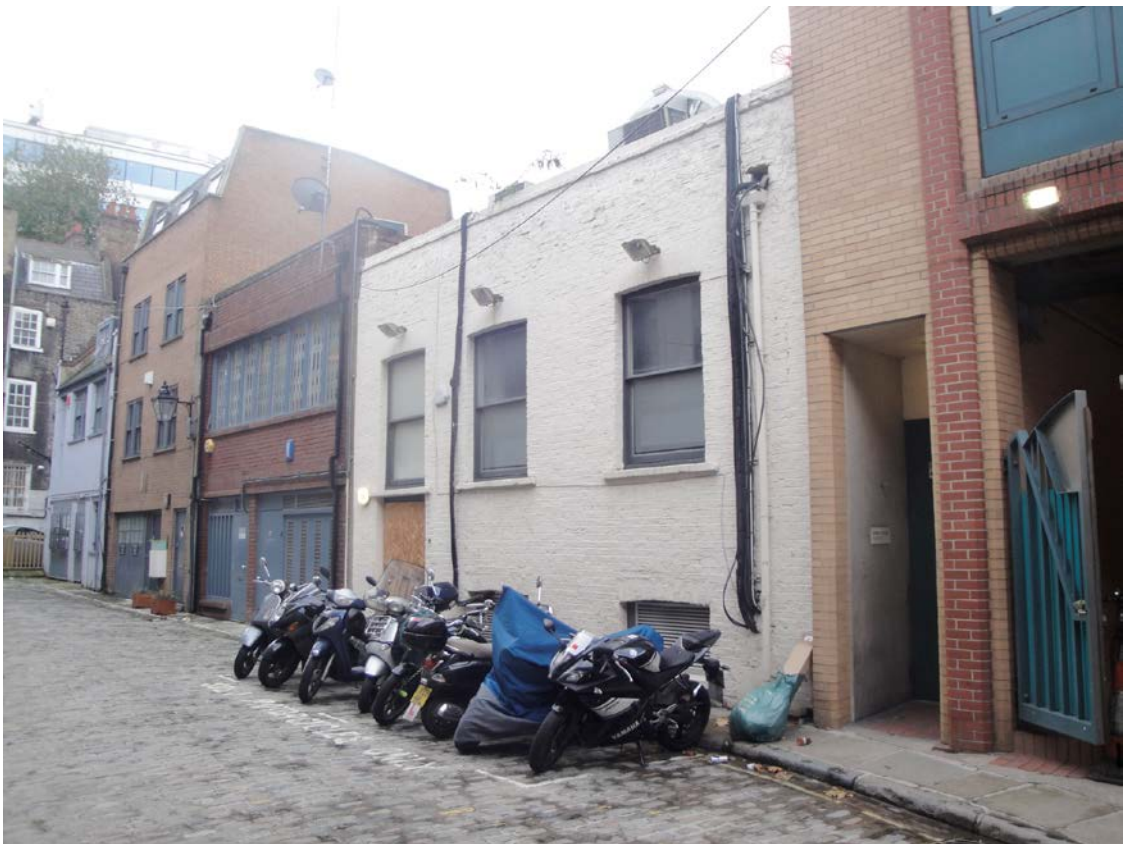
PHOTO 4 REAR OF 74 CHARLOTTE STREET
