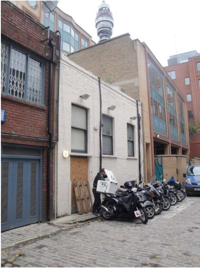
PHOTO 5 REAR OF 74 CHARLOTTE STREET
