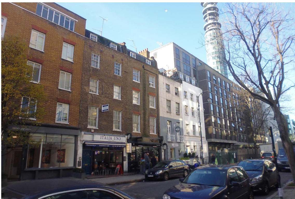
Figure 1. A view looking north along Charlotte Street, on the opposite side of the street from the application site.
