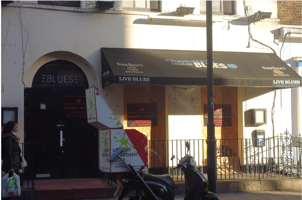
Figure 7. Detail of the ground floor entrance and frontage to Charlotte Street.
