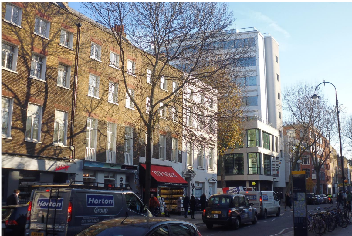
Figure 2. A view of the larger scale property on the corner of Tottenham Street and Charlotte Street.
