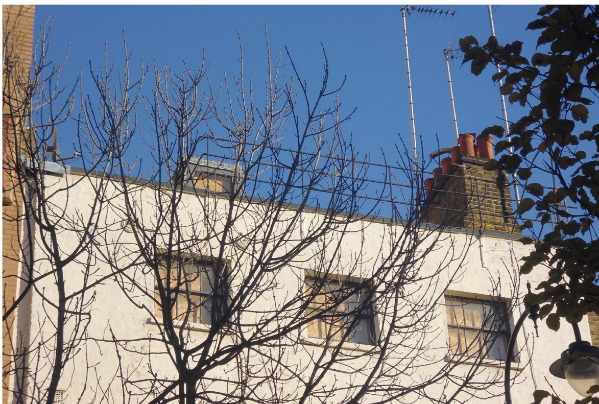
Figure 4. An image of the roofscape at 74 Charlotte Street.
