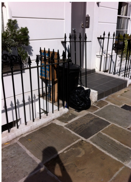
Neighboring Property's platform
