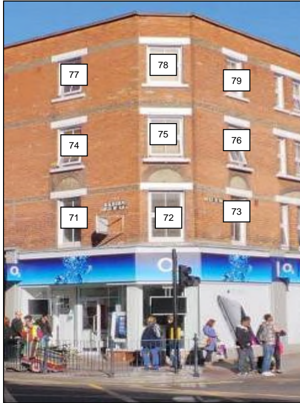
128 Kilburn High Road
