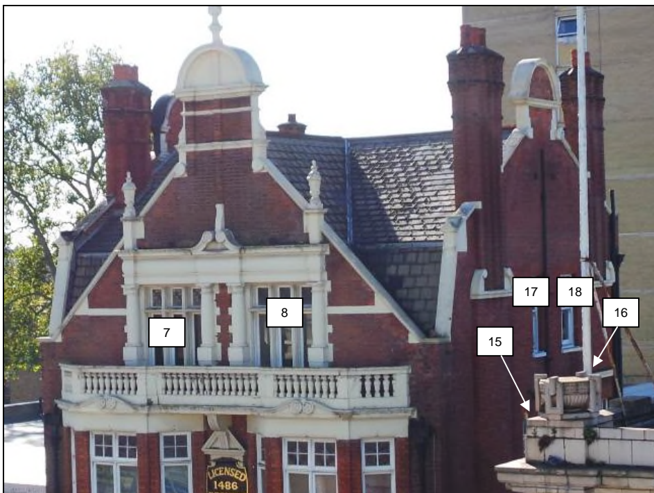
125 Kilburn High Road
