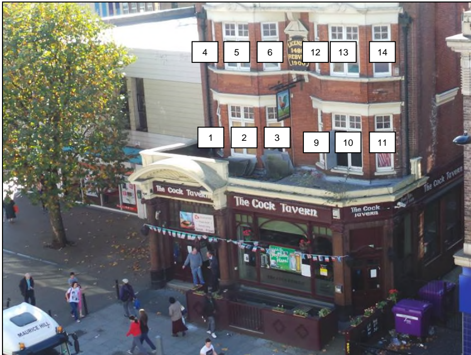
125 Kilburn High Road
