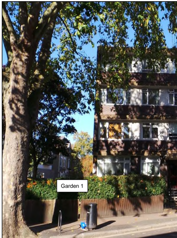
1 to 16 Daynor House
