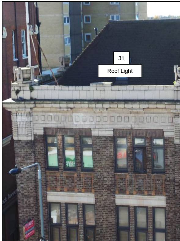
127 Kilburn High Road
