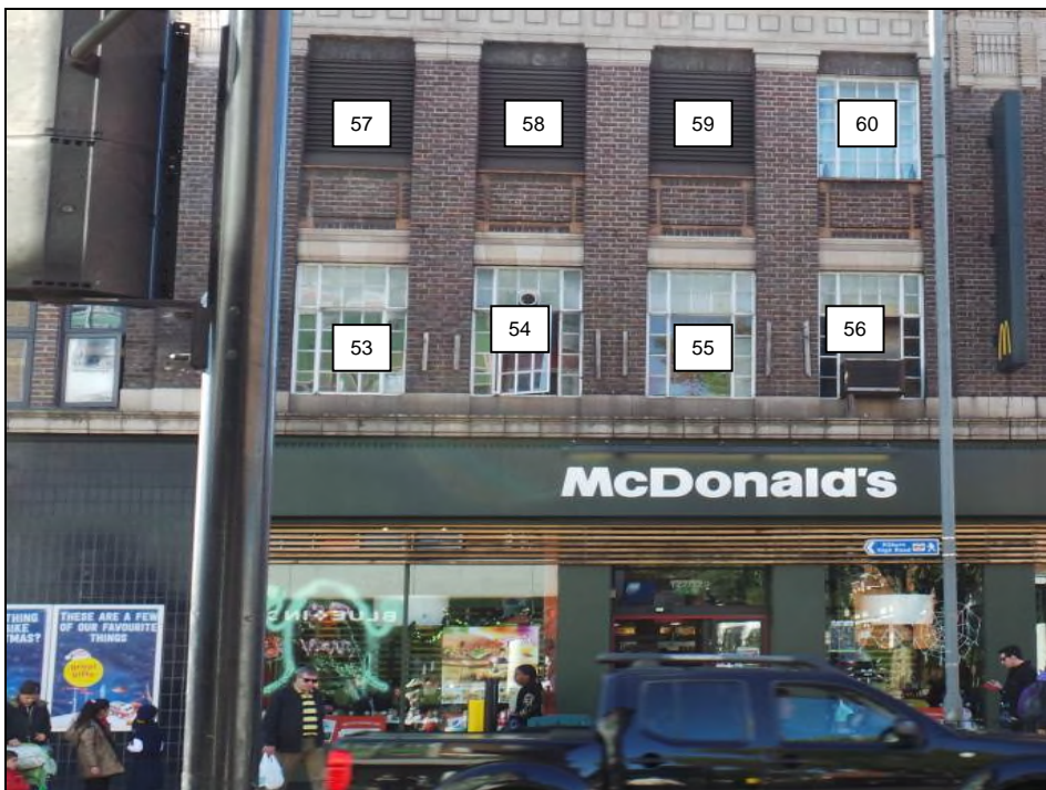
129 Kilburn High Road
