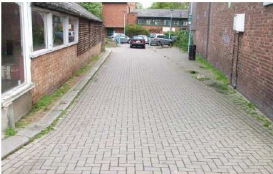
Photo 2 Shared access leading to Globe LTC with kerb to site and wedge shaped strip along south side Note 1 Timber bollards have been removed to wedge to facilitate parking. 2 Blue gate posts to Globe car park 3 Strip between kerb and shop is too small for pedestrian access.
