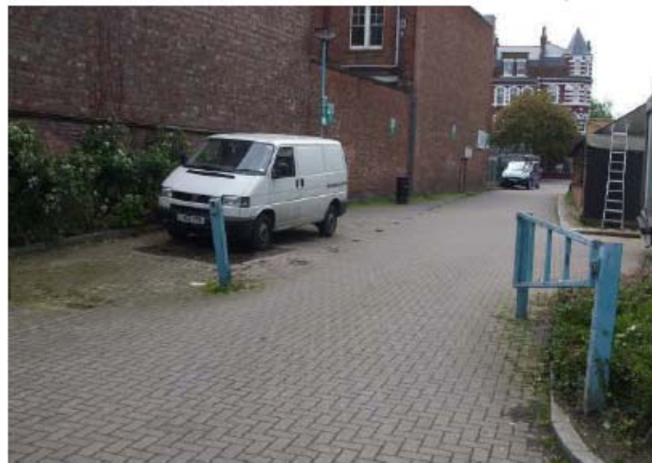
Photo 3 Rear of shared access with gate to Globe LTC car park Note 1 Illegally parked van on wedge shape and timber bollards cut down to ground level
