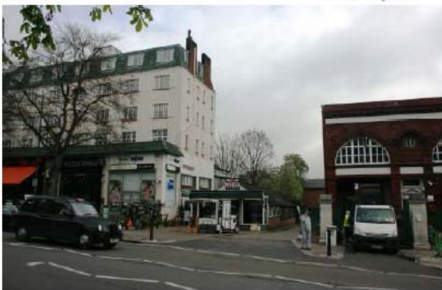
Photo 1 192 Haverstock Hill & shared access with Belsize Park Station to south and Aillingham Court to north Note 1 Zigzags to pelican crossing extend across shared access and the southern end of the site. 2 Bollard to shared access entrance which will need to be removed during the works.
