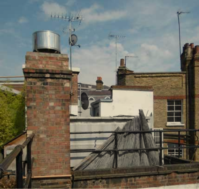
Existing water tank with poor quality lightweight screening
