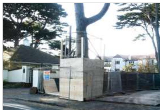
Photo 6: Board secured to scaffold framework adds another layer of protection for vulnerable trunks and branches.
