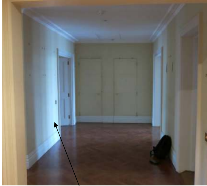
No.5 Entrance Hall with location of proposed lift
