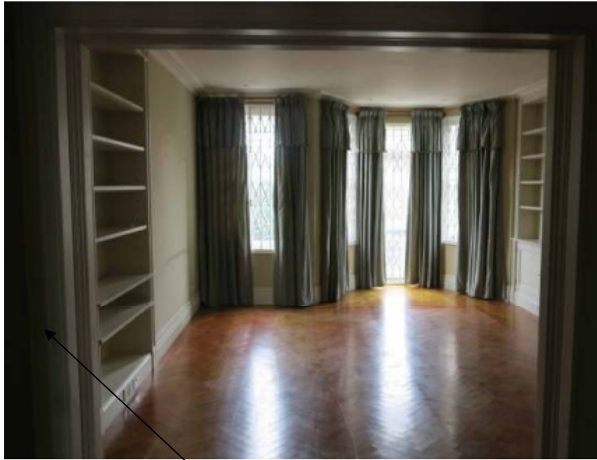
No.7 Partition wall to be removed between kitch and study at third floor
