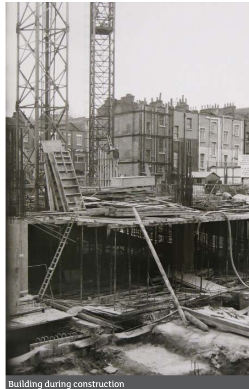
Building during construction
