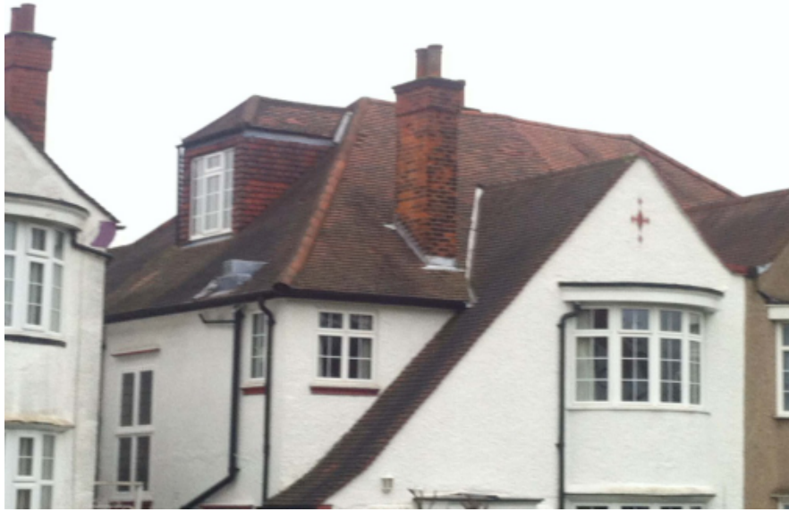
4HW side dormer
