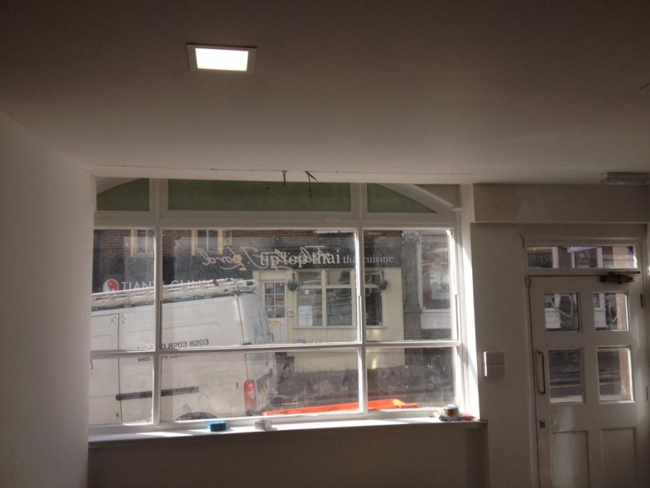
Photo taken 7 March 2014 showing bulkhead removed
